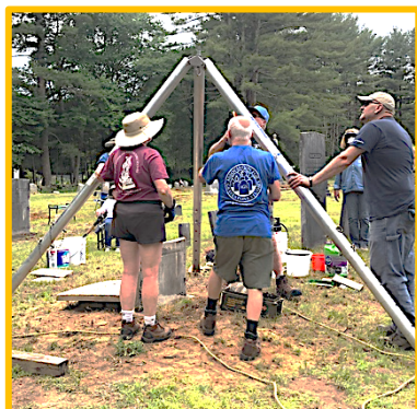
Andre Ribeiro and Rich Schofield assist as Betty and Carlo demonstrate the use of a tripod to lift large broken stone pieces into place.
